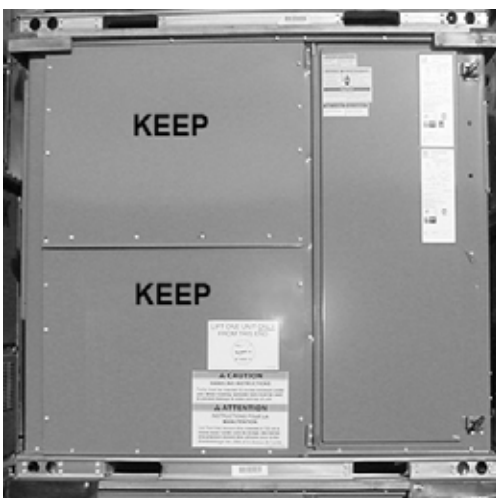
Figure 19: Save Side Panels For Economizer Hood Tops
